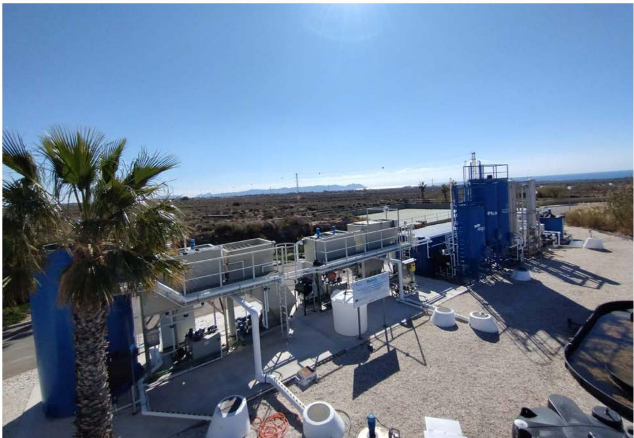
Aerial view of REUSA Hub.
